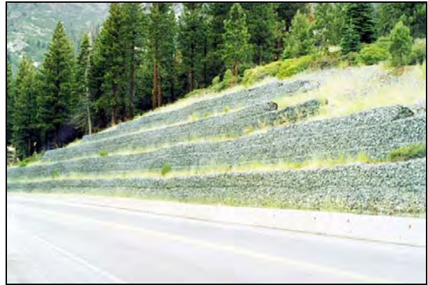
The rock gabion treatment of this hillside creates strong contrasts in line and color.
