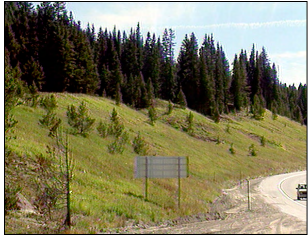
Rounding the top and bottom of the slope and also undulating the face of the slope create a more natural-looking landscape.
