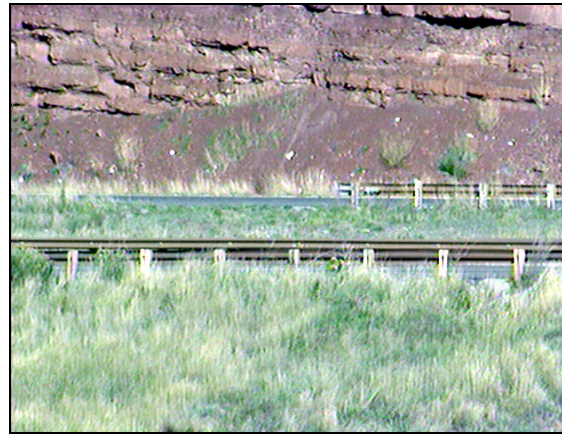
The color of these guard rails is appropriate because it creates very little visual contrast.
