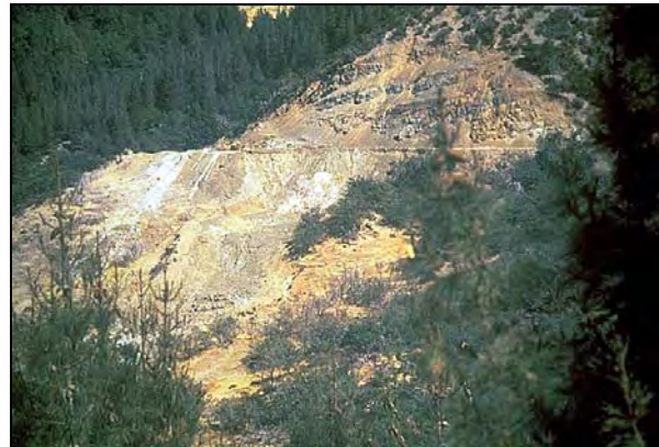
Downslope wasting of excess material dramatically increases the size of the visual scar.
