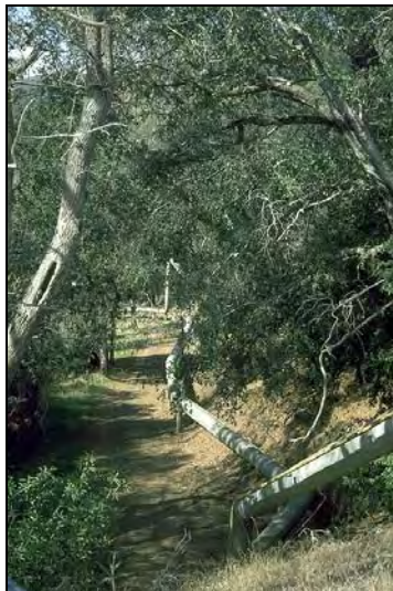
Creative pipeline alignment.
