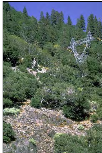
Transmission tower (left) painted to blend with vegetation.
