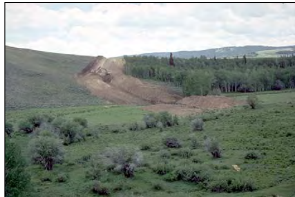
This pipeline location avoids the wooded area and minimizes disturbance.
