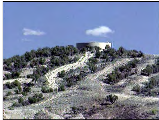
This water tank is set back from the crest of the hill, thereby reducing the visual impact; however, the access road could have been better located.
