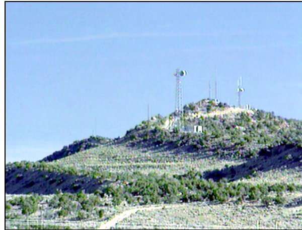
Consolidation of communications facilities reduces the Amount of visual sprawl.
